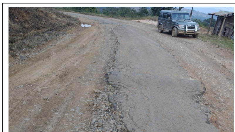
PHOTO: POOR ROAD CONDITION ON THE WAY TO SAIPUNG
